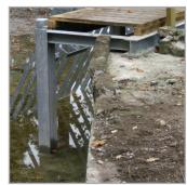
Stonbury were engaged to fabricate and install a new weed rack as part of the Environment Agency WLMP programme at Bodenham, near Salisbury. The weed rack was fabricated to EA specifications inhouse.
