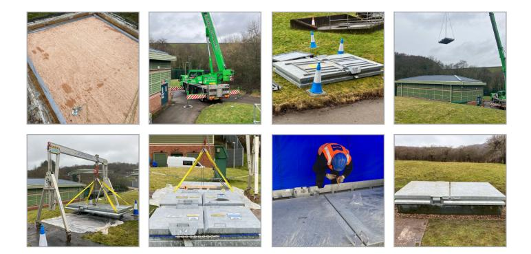
Stonbury was contracted to replace the hatch covers on a live potable water reservoir in the East Midlands.
