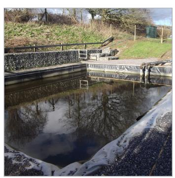
A final settlement lagoon required repair and refurbishment work due to wildlife damage and bank slippage, which had caused the lagoon to leak.
