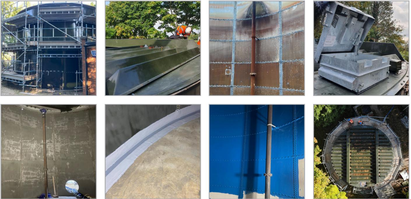
Stonbury was contracted to refurbish and replace the roof on an above-ground, modular bolted glass-fused-to-steel (GFS) tank.
