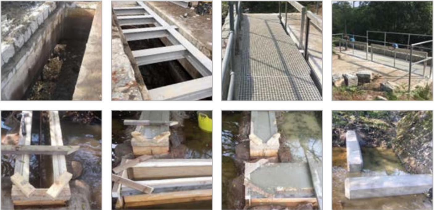
Stonbury was contracted to carry out modifications to an intake located on an impounding weir and off-take structure. The intake was used to abstract water from the catchment and divert it to a nearby raw water reservoir via a 42-inch underground pipeline. However, the structure was failing to effectively screen river gravel, debris and fish from entering the pipe.
