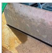
Stonbury is pleased to roll out the application of cutting-edge neoprene gasket seals, a new WRAS-approved alternative to mastic for sealing treated water asset hatches.
