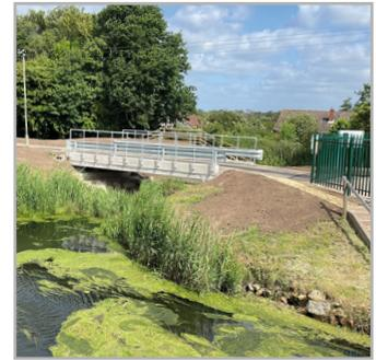
A specialist Stonbury team was deployed to undertake the replacement of a bridge for the Environment Agency. After an inspection, the existing bridge had been downrated to a maximum weight allowance of 3 tonnes which was unsuitable to allow access of vehicles to the nearby pumping station.
